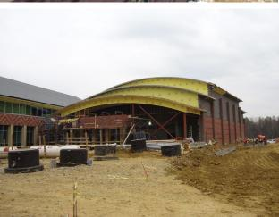
Construction of a new three-story, 188,440 GSF, high school for the Diocese of Arlington VA near the Potomac River in Dumfries, VA. Project is a steel frame structure with masonry and cold-formed metal frame (CFMF) backup walls protected by air and weather resistive barriers and primarily clad with brick veneer and exterior insulation & finish system (EIFS). Glue-laminated timbers are incorporated at several of the vaulted roof structures.
