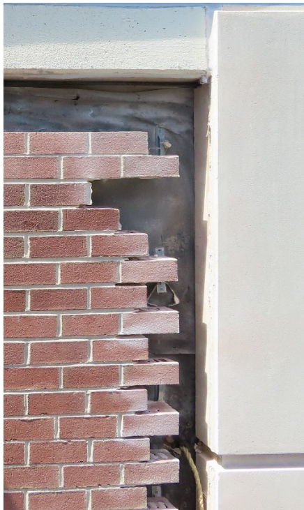
CONVENTIONAL VERTICAL BRICK TOOTHING
