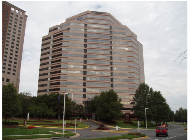
1650 Tysons Boulevard, McLean, VA 391,300 sf, 17 stories plus basement and an adjacent 5-level parking structure
