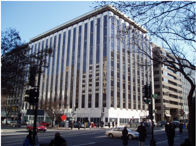
1776 K St. Office Building, Washington, DC 291,150 sf, 12 stories plus 3 levels of parking
